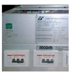
For the substation SECOM developed natural air cooled power rectifier at 3000 Vcc to fed the eletrical line network while special protection devices are installed along the railway tracks to avoid sudden and dangerous overvoltages SECOM also developed switching power supplies with high
